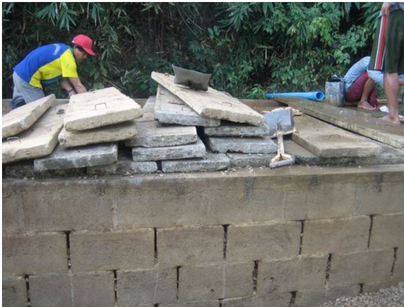
Figure 3-7: Internal wall of SP-10 HFRF.
